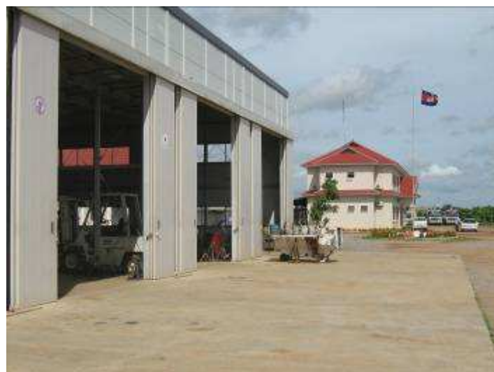
Everything is well equipped at CMAC which is mostly donated by other countries
