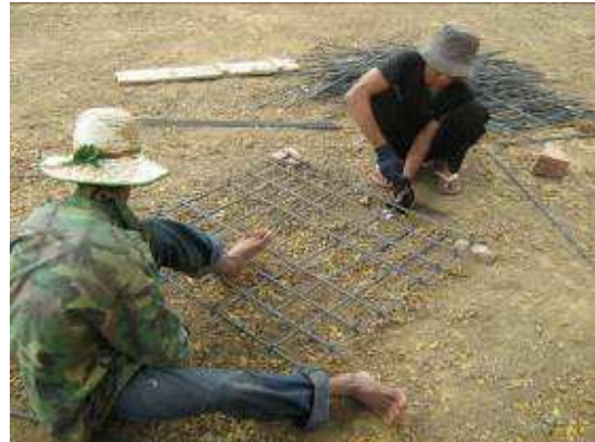
The workers are preparing the next step: nettings for the cement.
