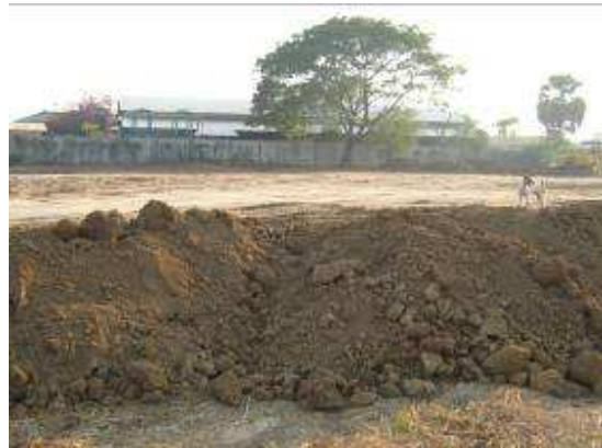
To avoid later flooding by heavy rainfall the land is filled up by 1 m in height
