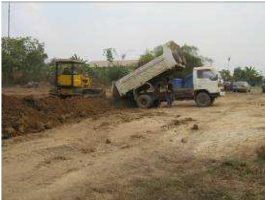
To avoid later flooding by heavy rainfall the land is filled up by 1 m in height
