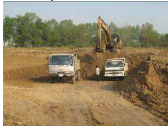
The old pond is filled with earth from where the place of the new pond
