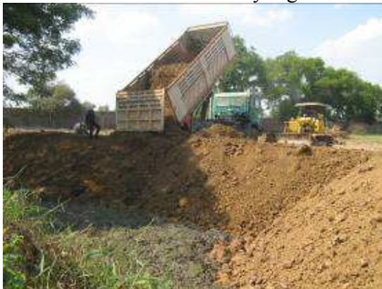
The old pond is filled with earth from where the place of the new pond
