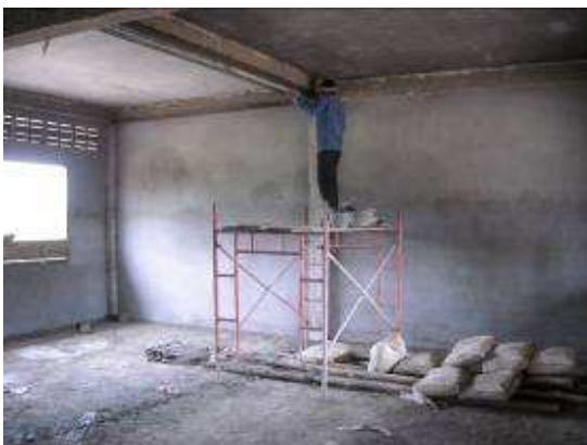
In the meantime on the groundfloor the walls are getting plastered.
