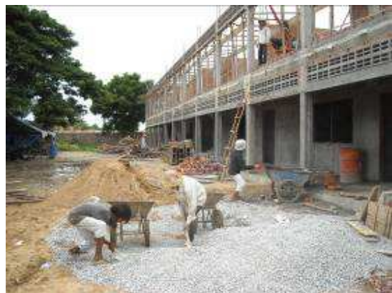
In the meantime on the groundfloor the walls are getting plastered.
