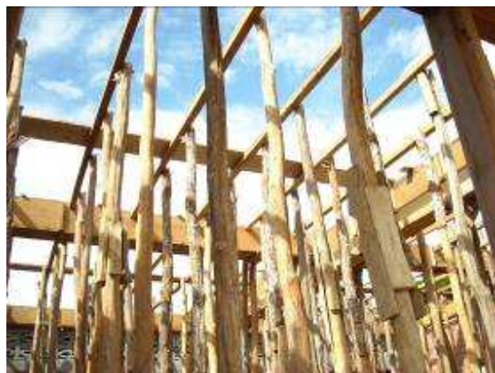
Support beams for the construction of the first floor
