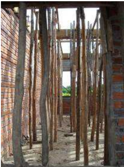
Support beams for the construction of the first floor
