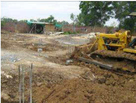
The holes for the foundation poles is closed with earth
