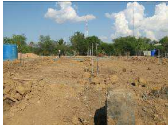
The holes for the foundation poles is closed with earth
