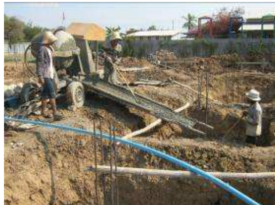
Cement is mixed and used for the foundation.
